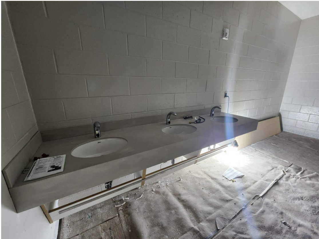
Sink install in progress in gang bathroom.
