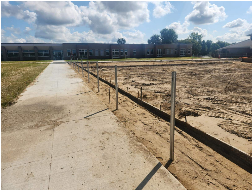
Concrete walks formed and fence poles installed at 2nd grade playground on the west side of the building.
