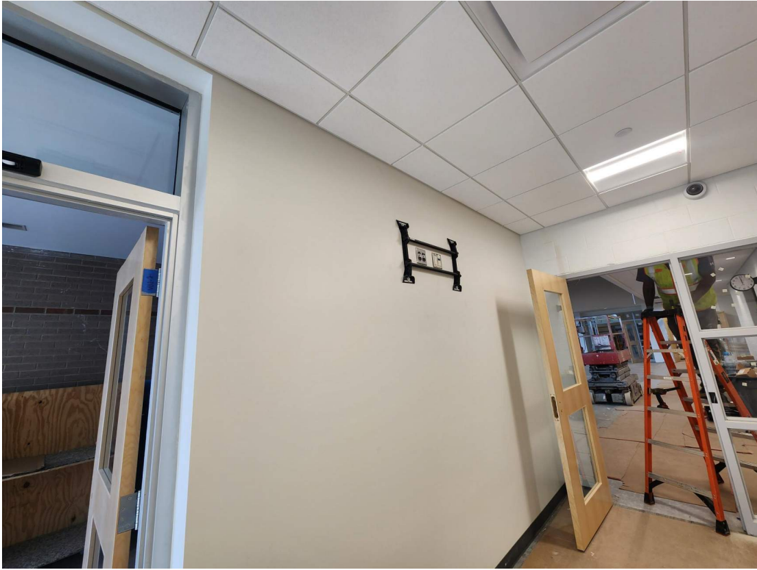
Display mount installed in reception.
