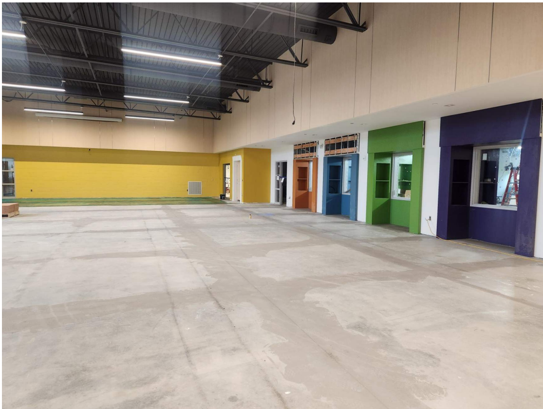
Wall covering and plastic laminate installed in cafeteria.
