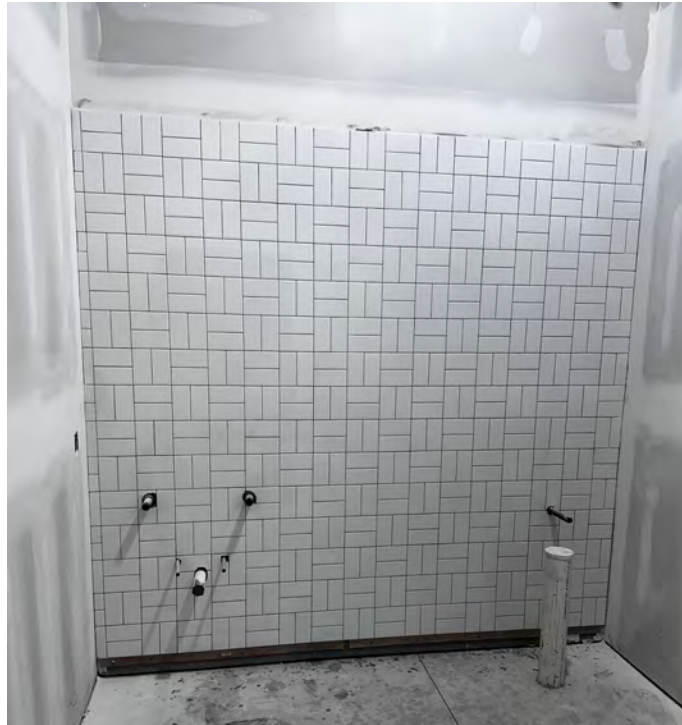
Wall tile completed in office bathroom.
