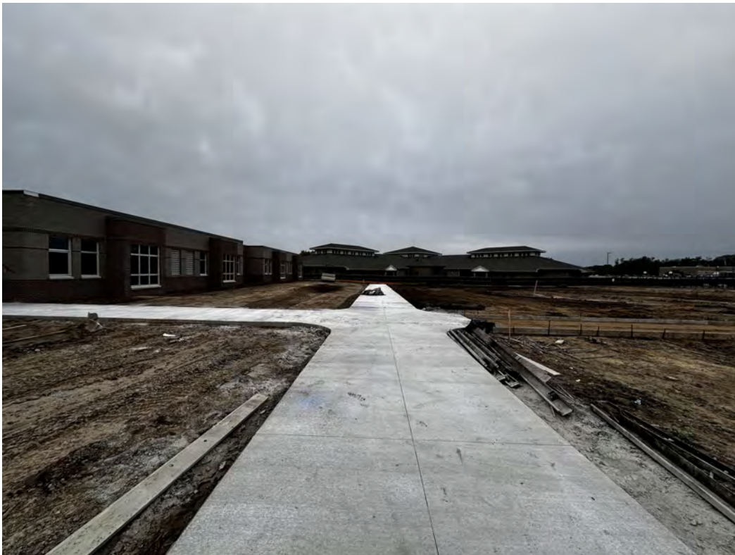
Concrete walks on west side of the building.
