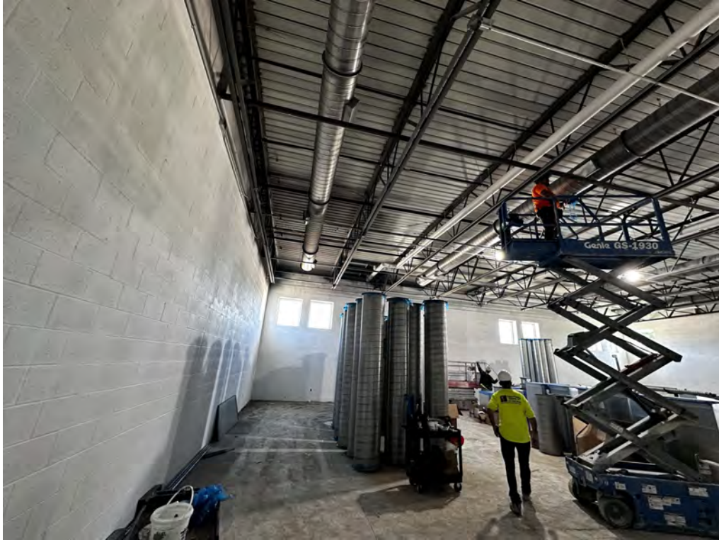
Gym duct install in progress.
