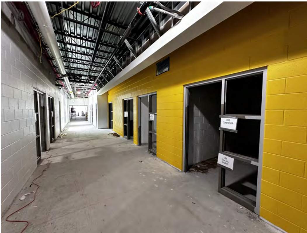
Painted hallway walls in center of the building.
