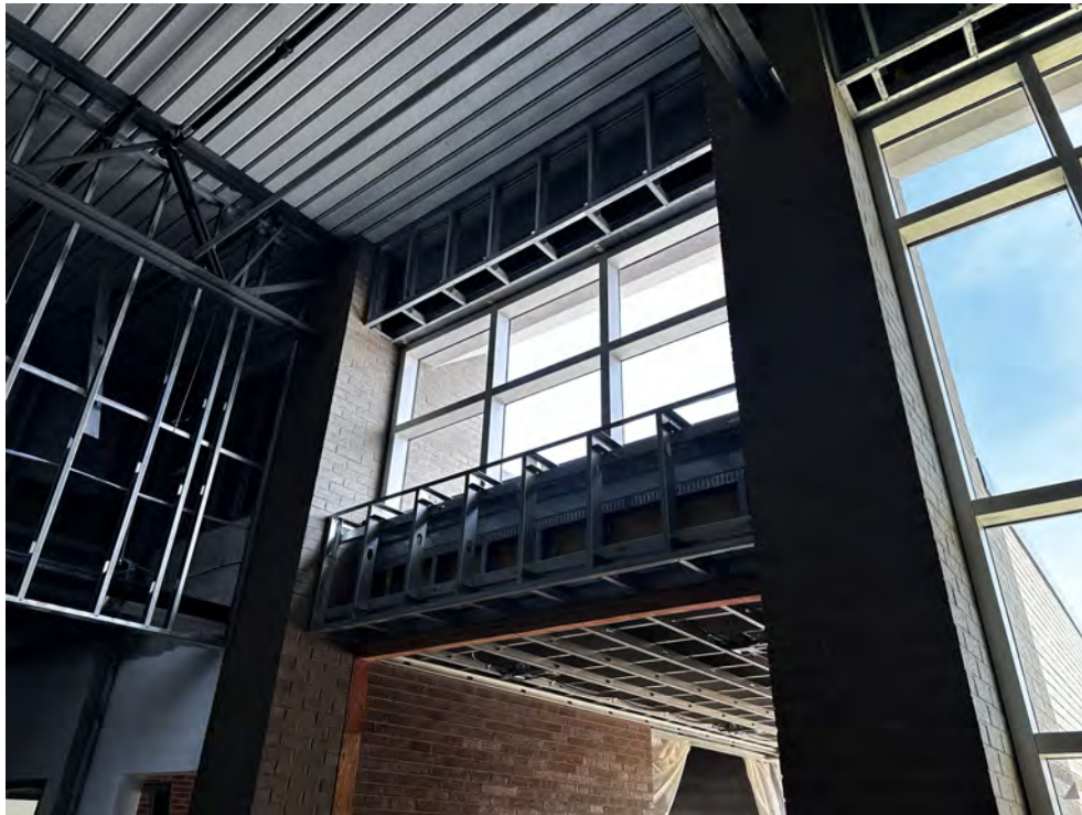
Vestibule window frame installed.
