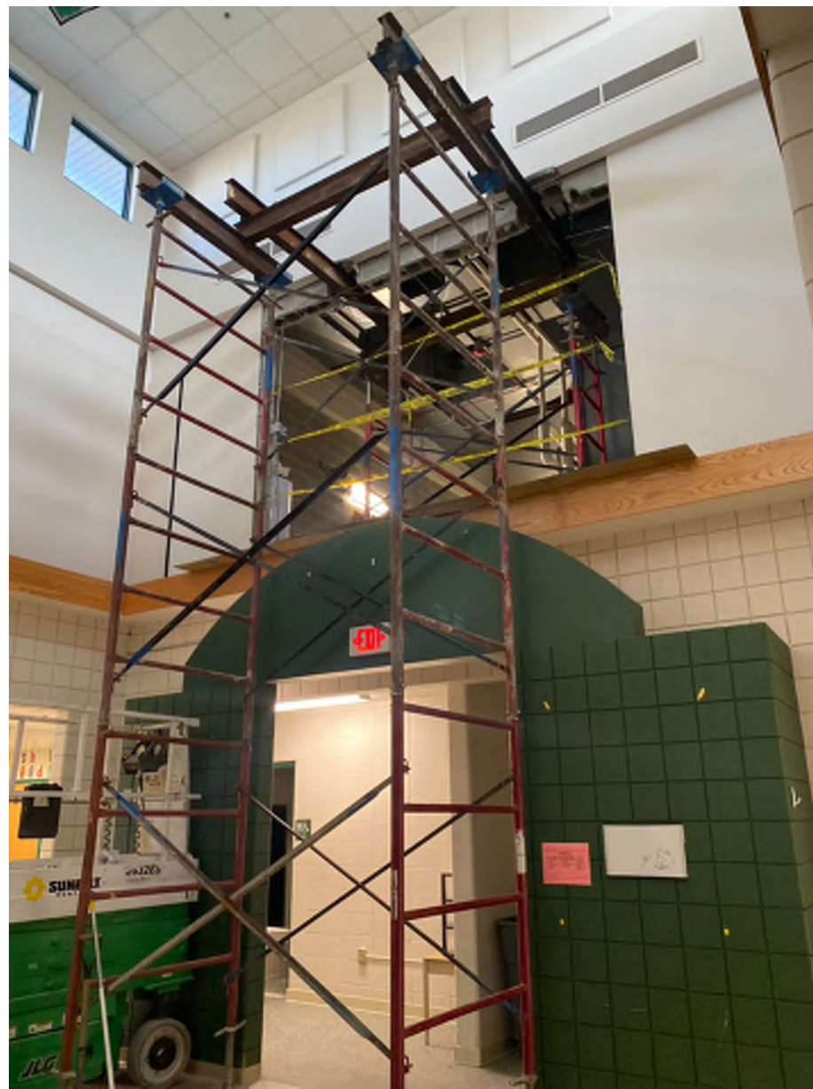
Scaffolding at mezzanine for demo of the wall opening.
