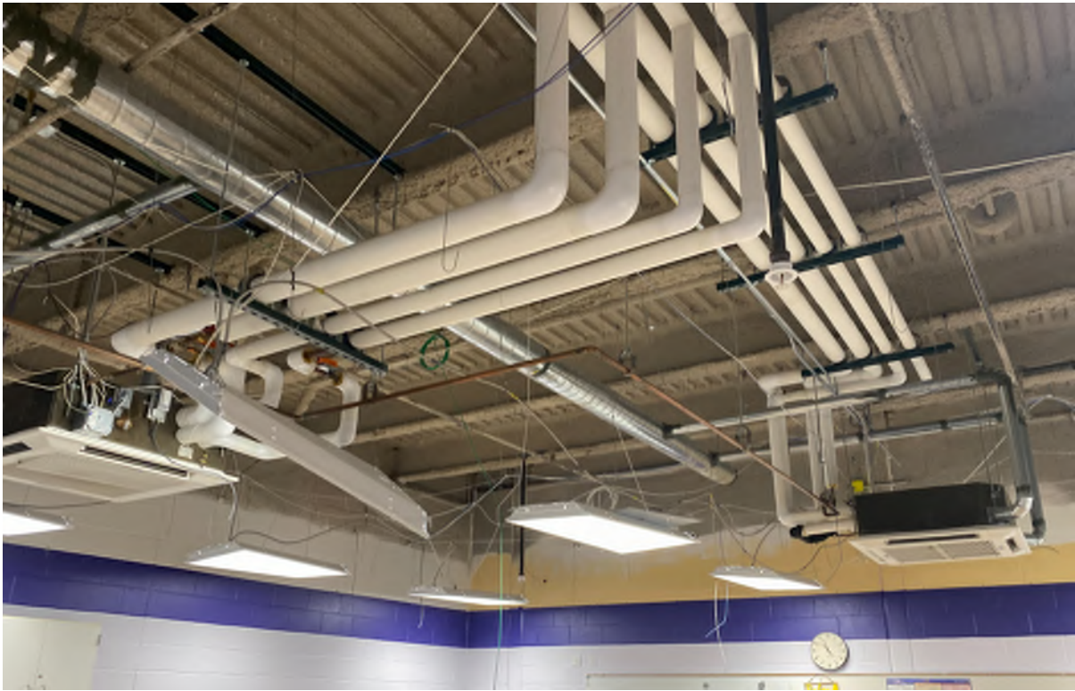
Pipe insulation at ceiling.
