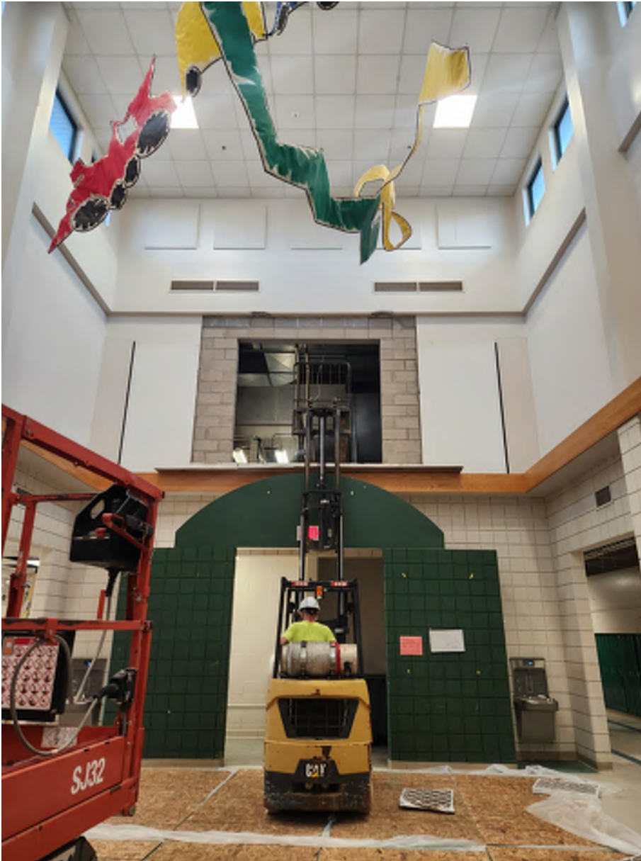
Mezzanine wall opening after demo in preparation for new mechanical equipment.
