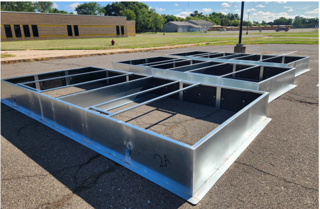
Rooftop unit curbs staged for install.
