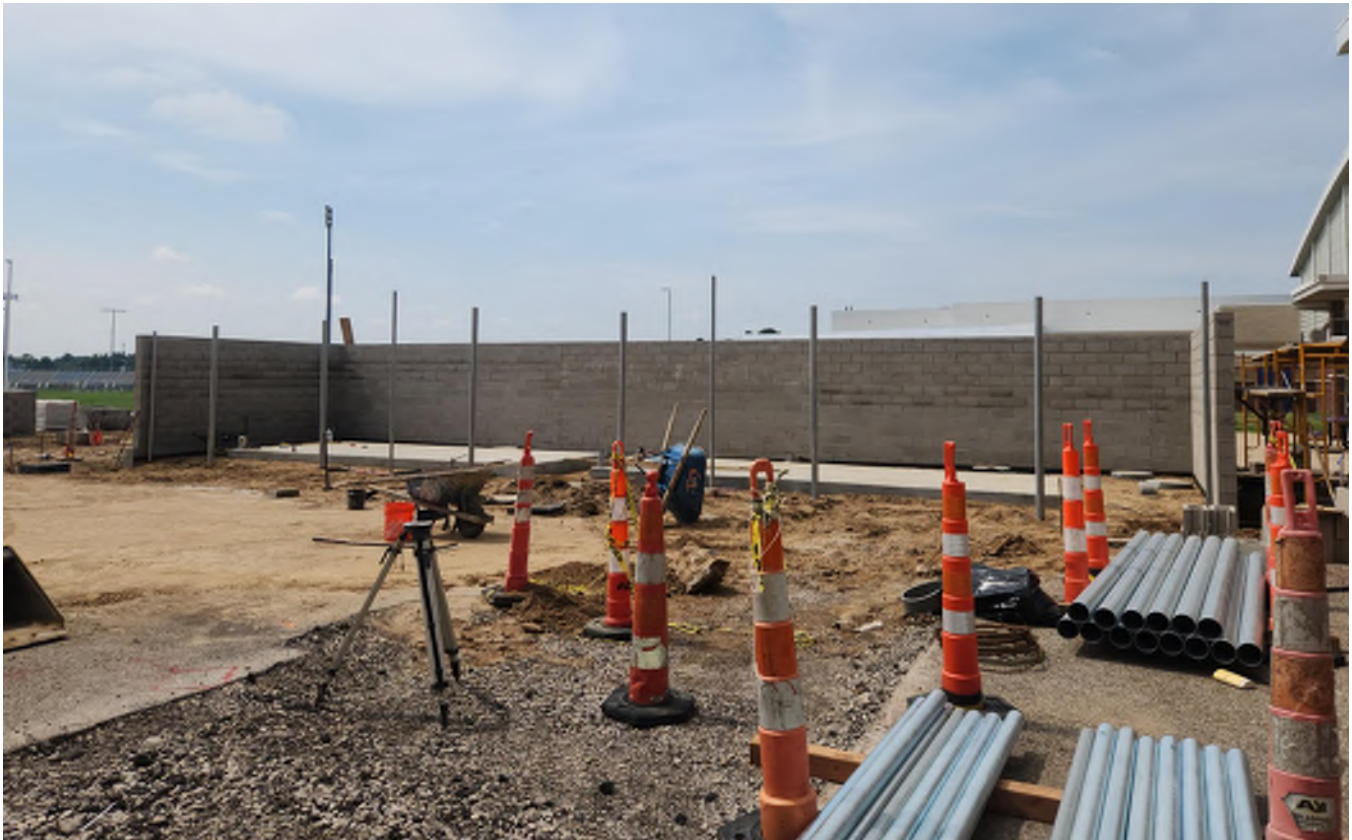
Chiller enclosure progress including concrete masonry units and fencing poles.
