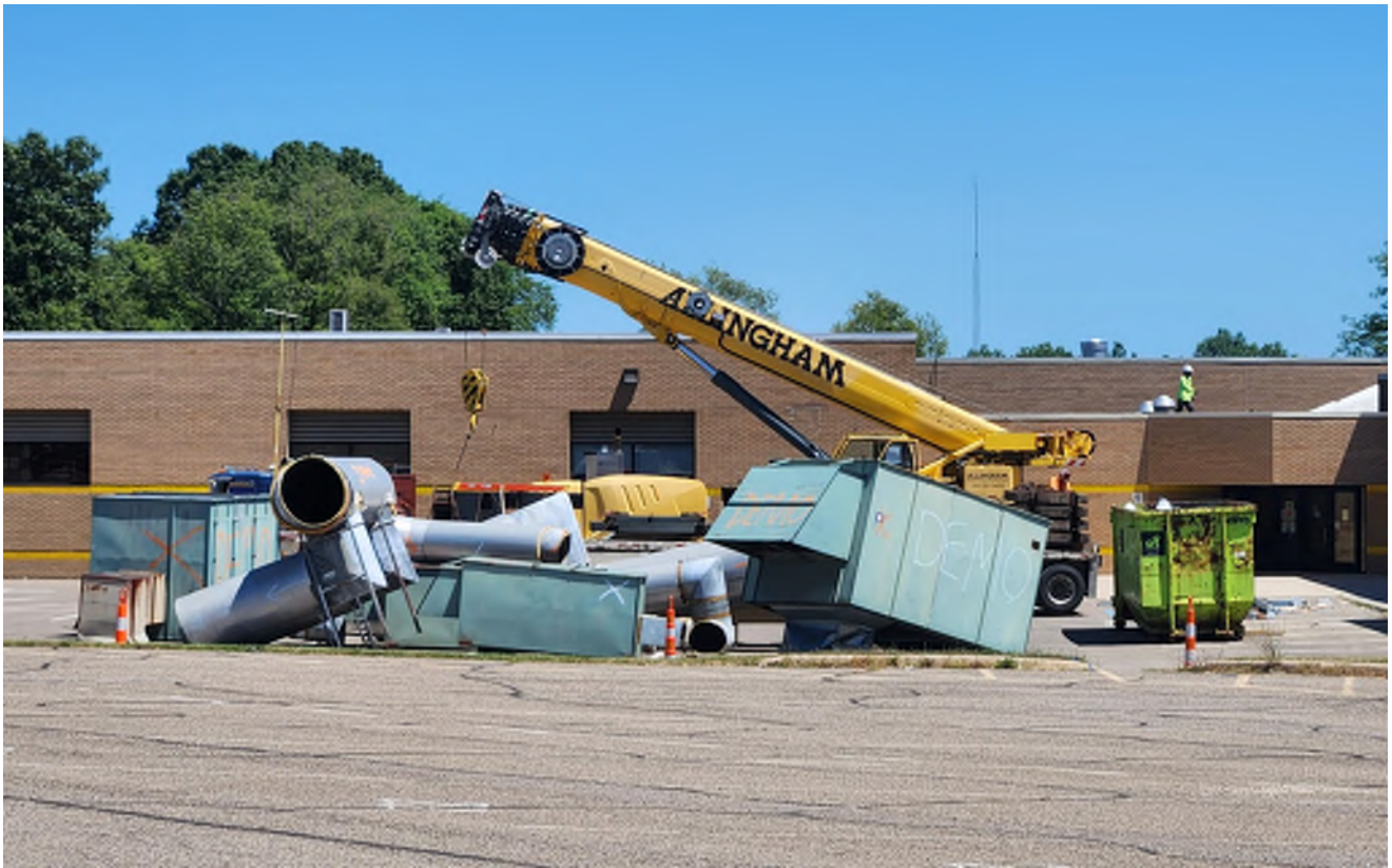
Demoed rooftop mechanical equipment.
