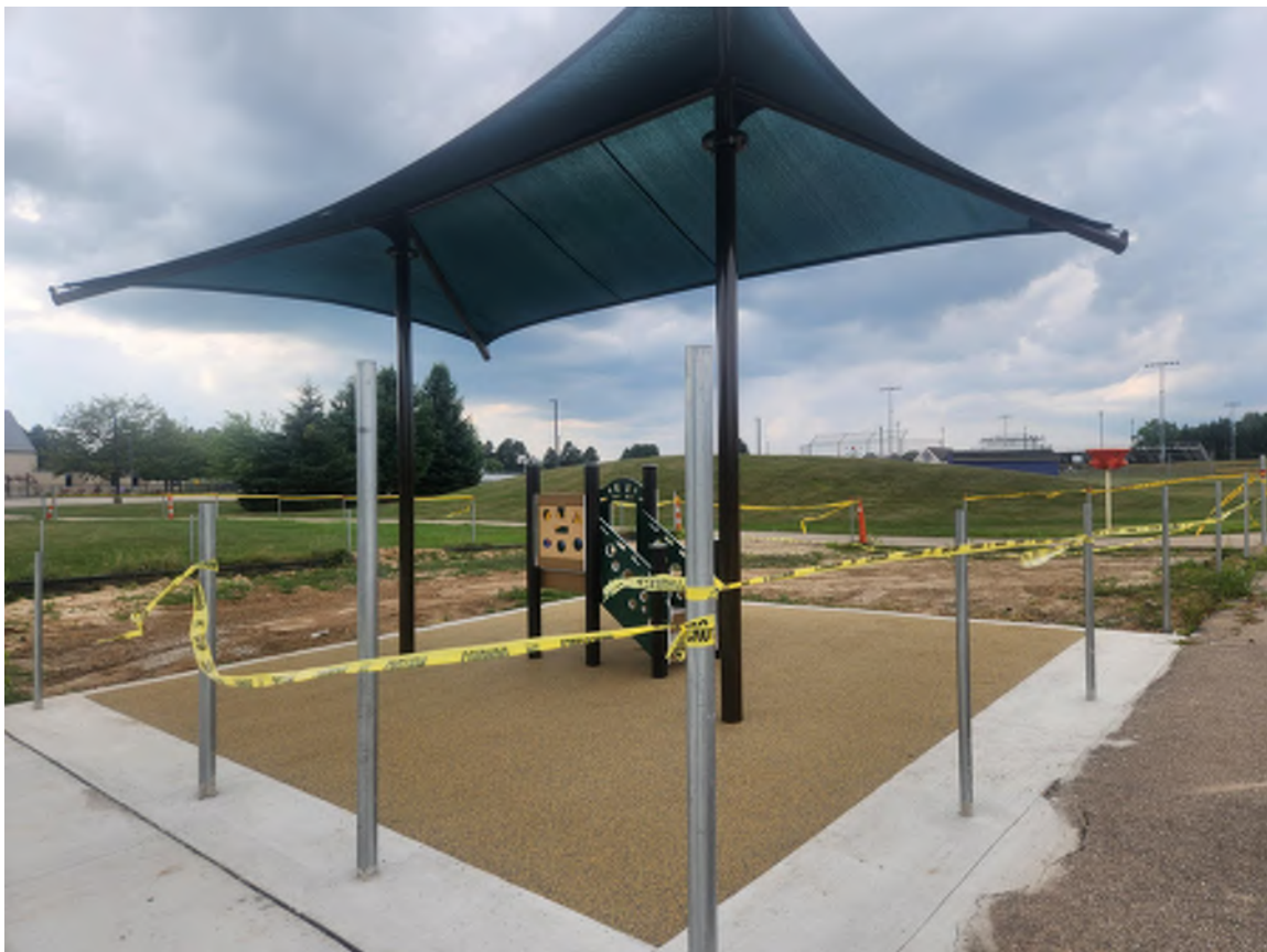
Shade and pour-in-place safety surfacing in toddler playground area.
