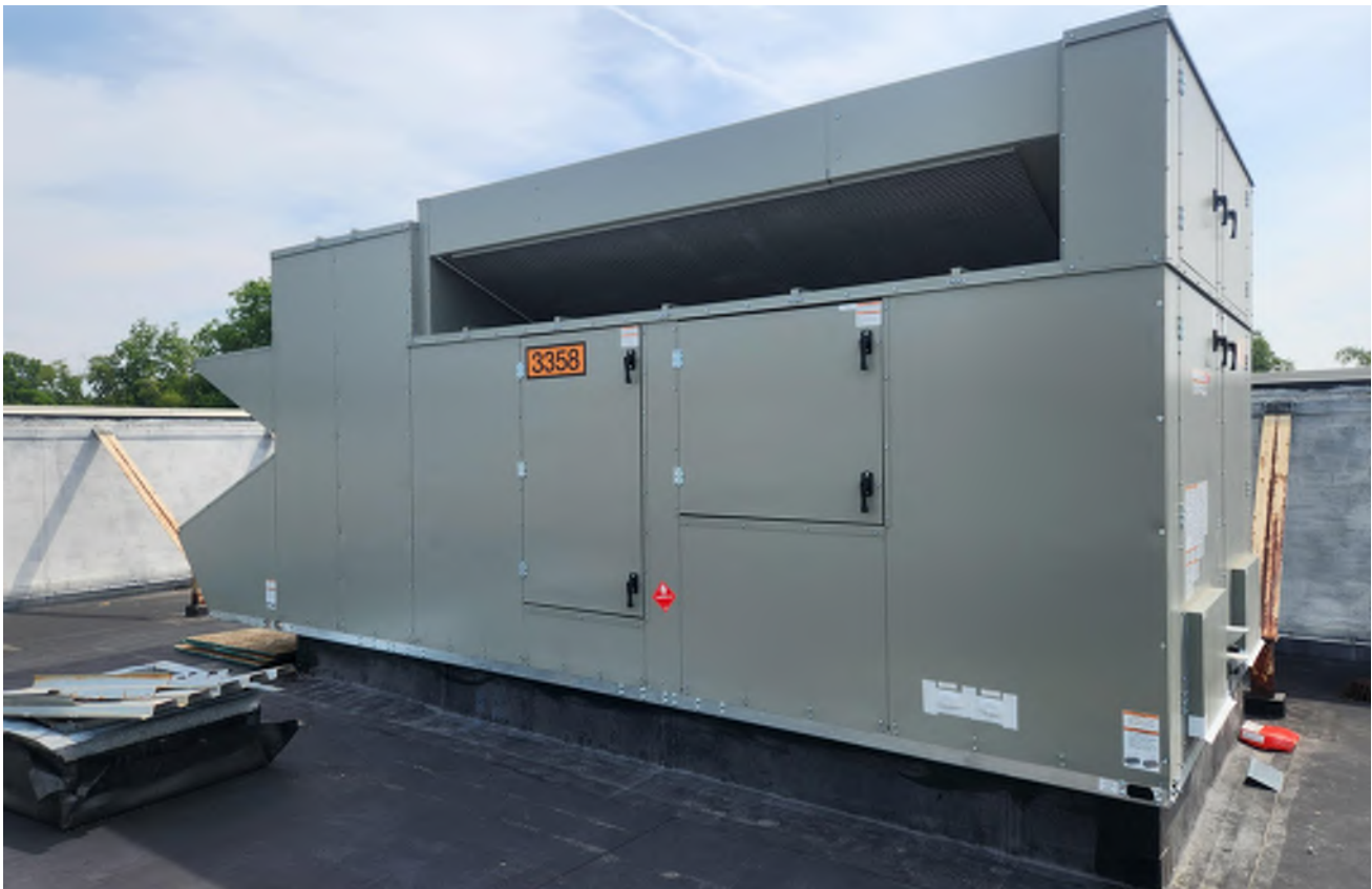
Two of the seven new rooftop units set on the roof.
