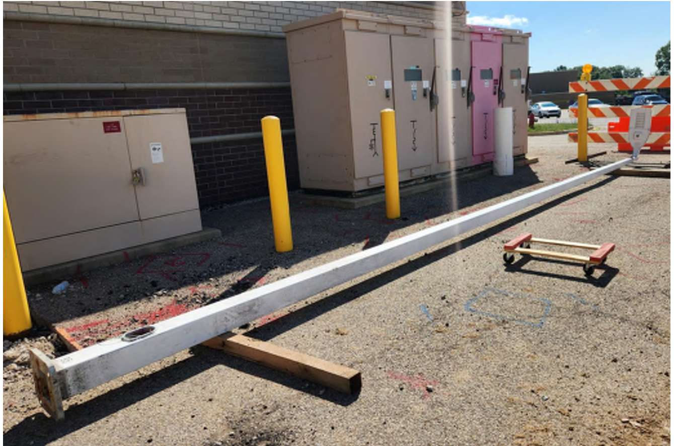
Demoed light pole after removal.
