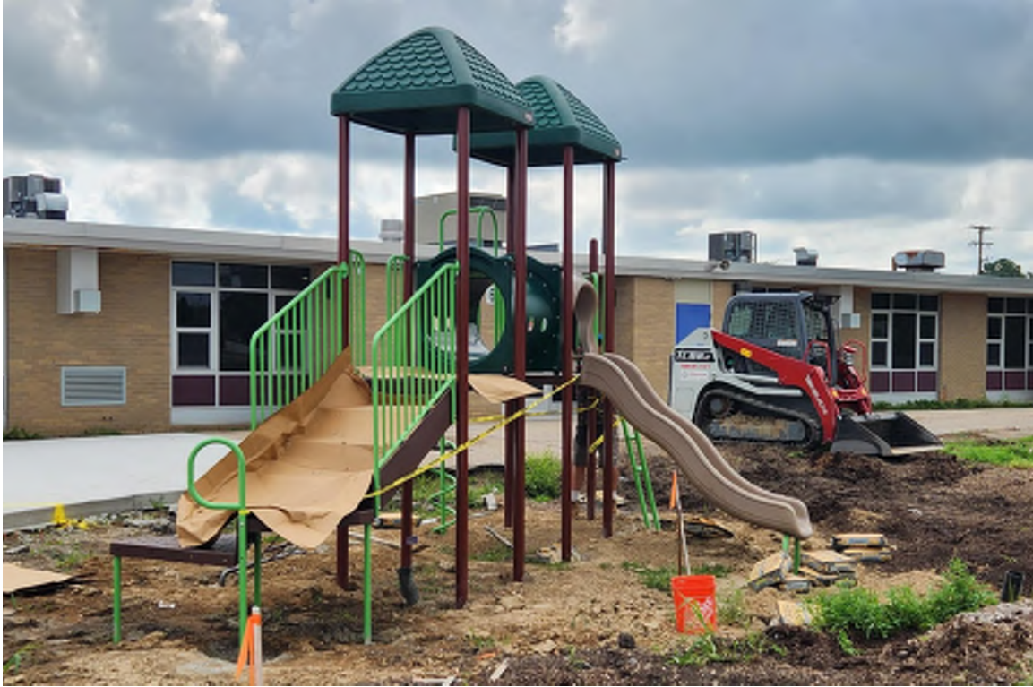
Age 2-5 playground equipment installed.
