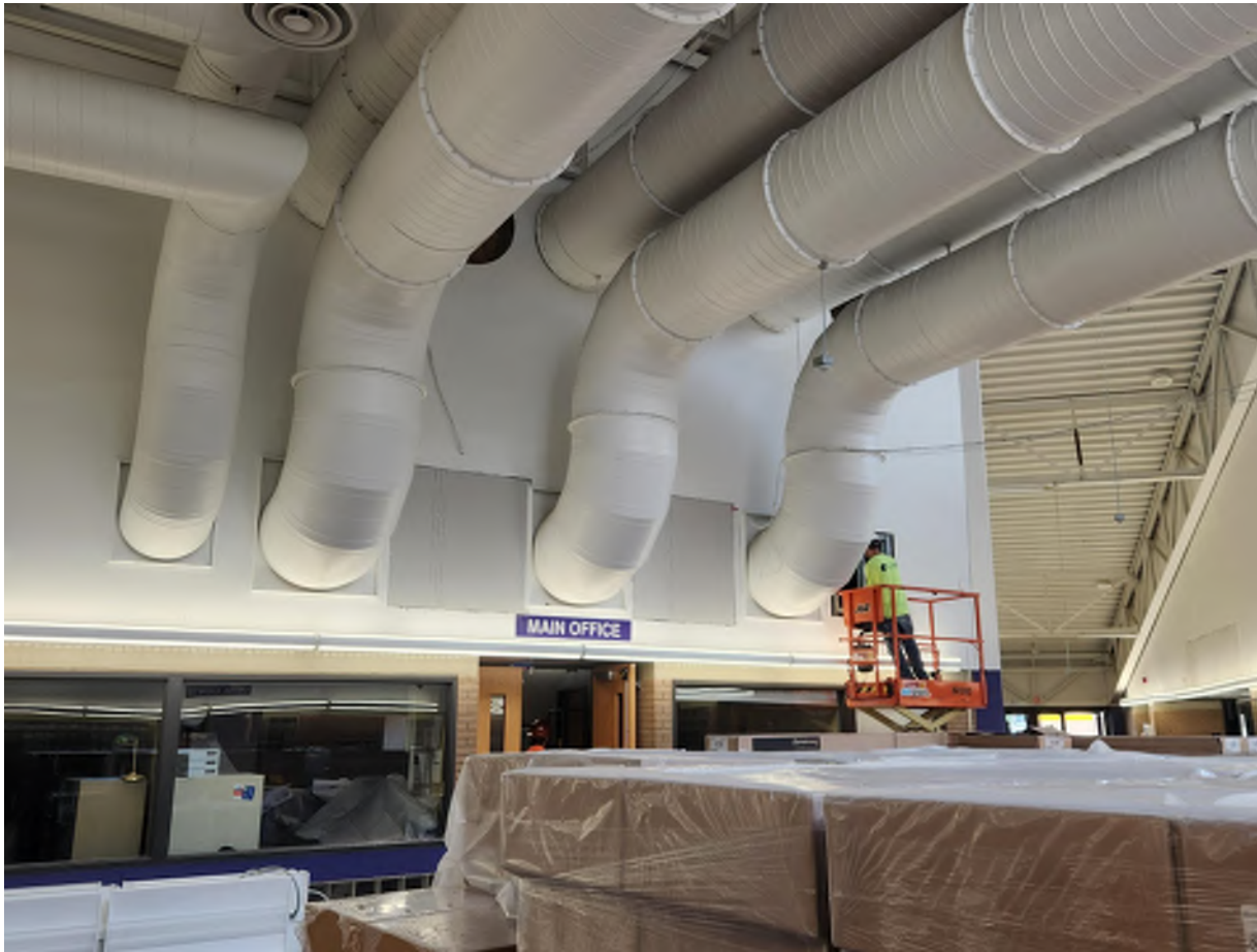
Duct openings being infilled with drywall.
