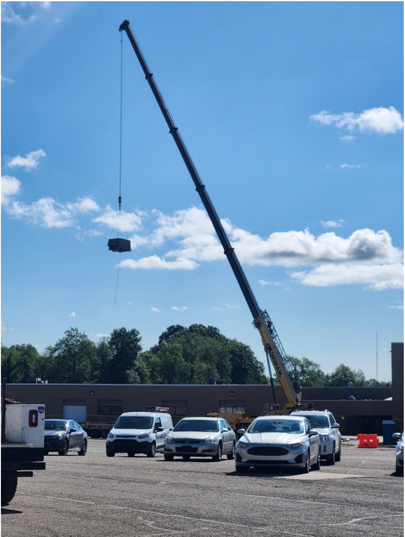
Demoed rooftop equipment being lifted by a crane.
