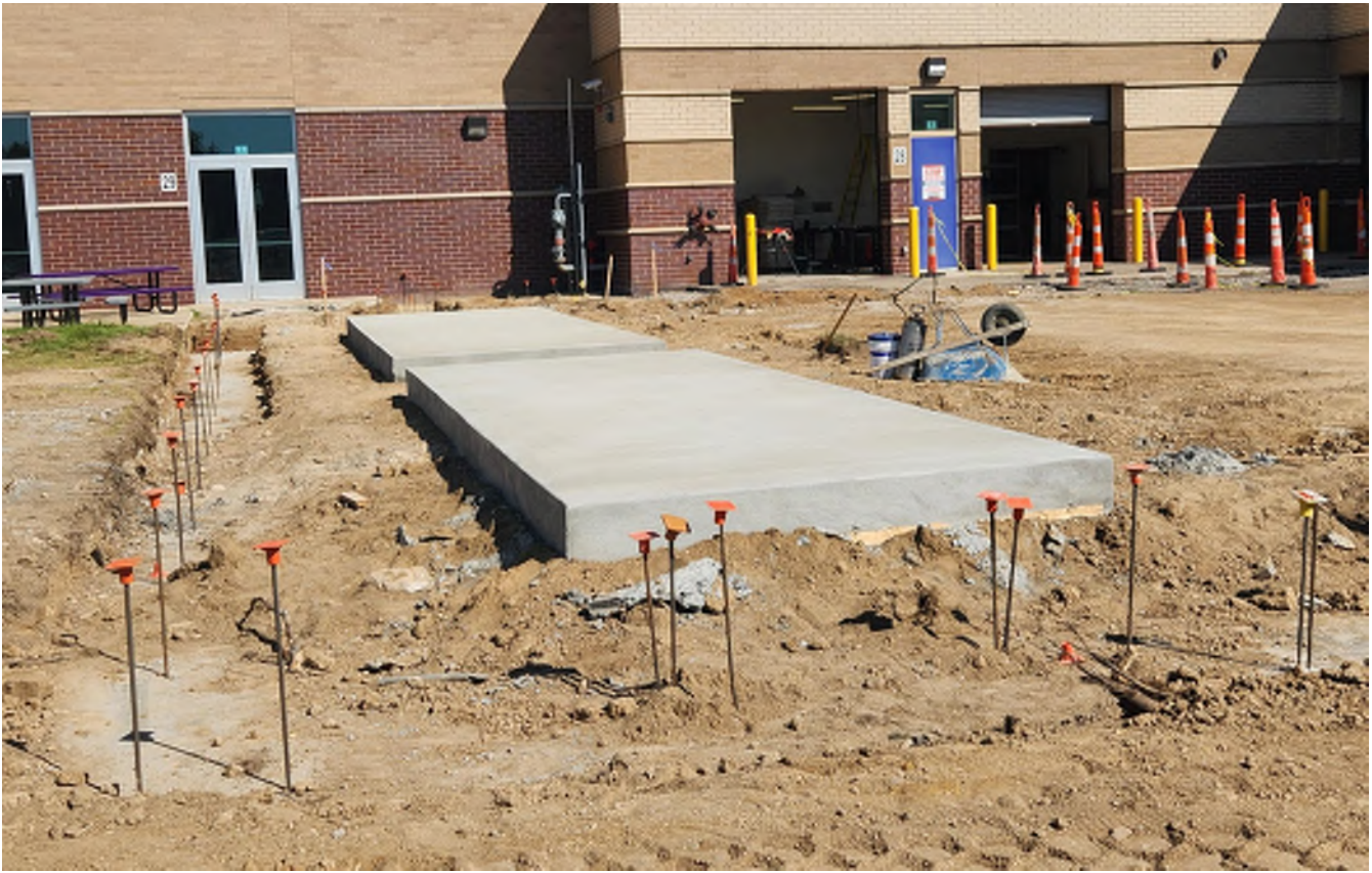
Chiller pads in preparation for enclosure and equipment setting.
