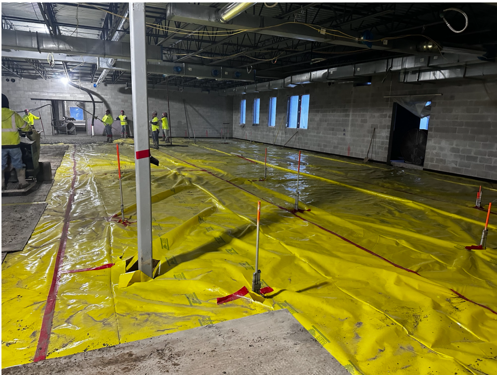
Vapor barrier laid down in preparation for pouring concrete.
