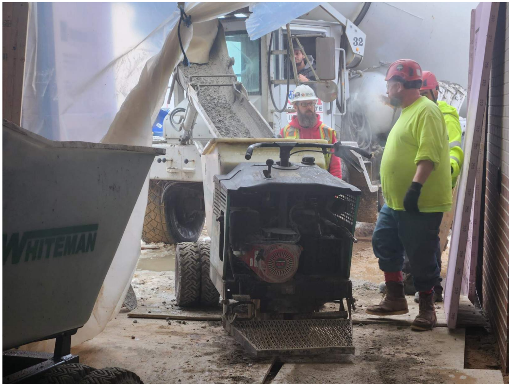
Concrete truck transferring concrete to a buggy.
