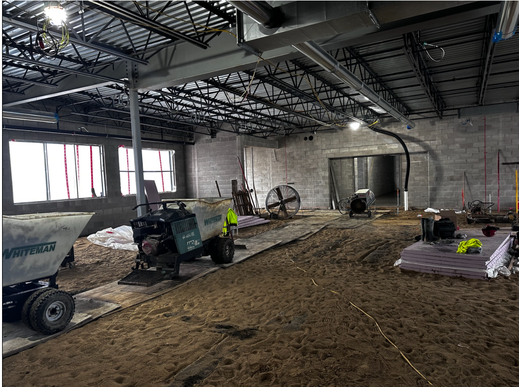
Buggies and boards laid out in preparation for pouring concrete.
