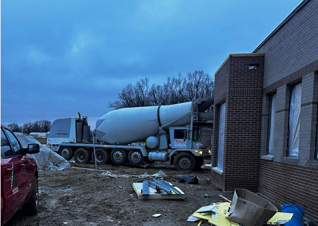
Concrete truck delivering concrete to west sided of building.
