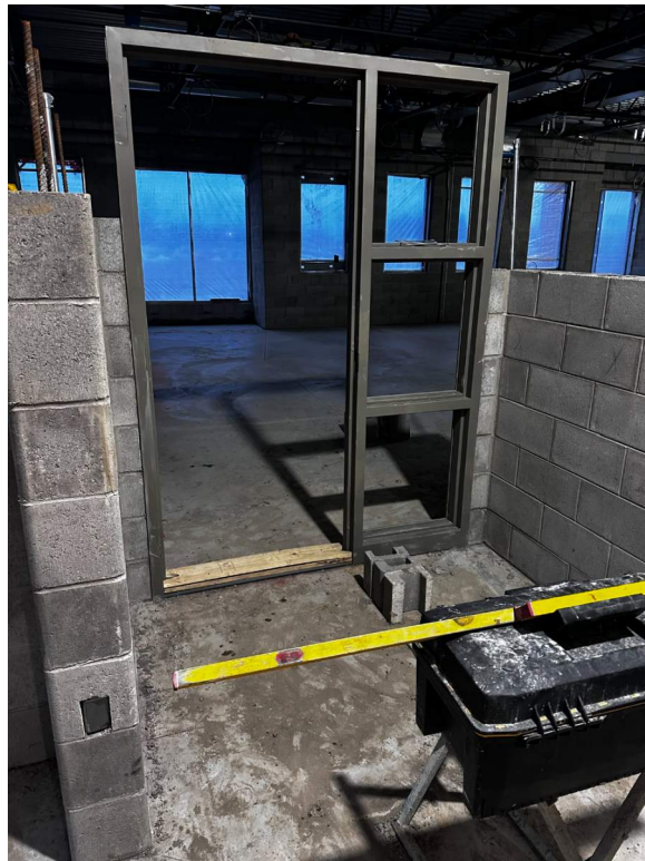
Hollow metal frame being installed in entryway.
