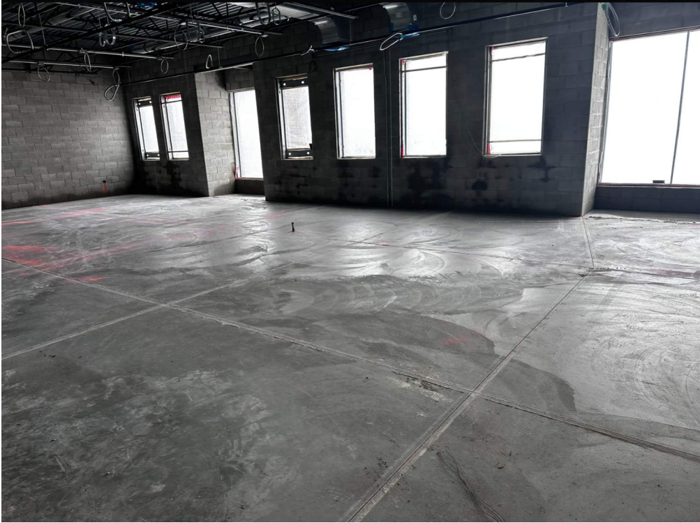
Slab after sawcutting in classroom.
