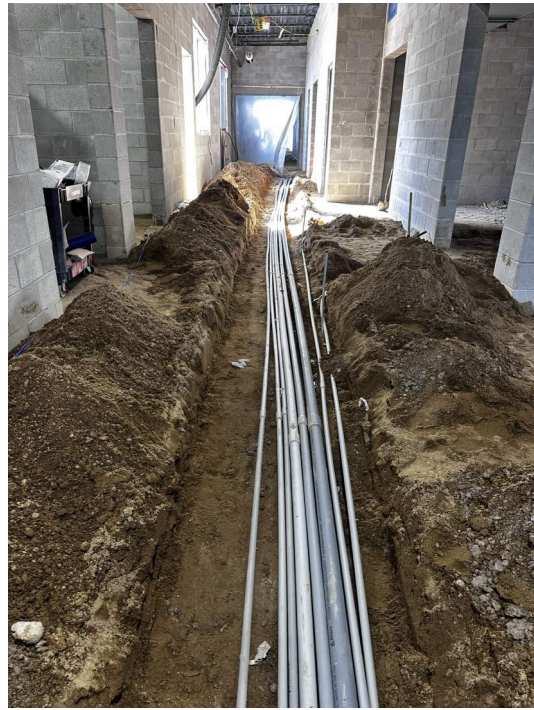
Electrical conduit install in hallway.
