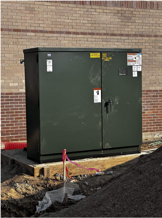
Transformer installed.
