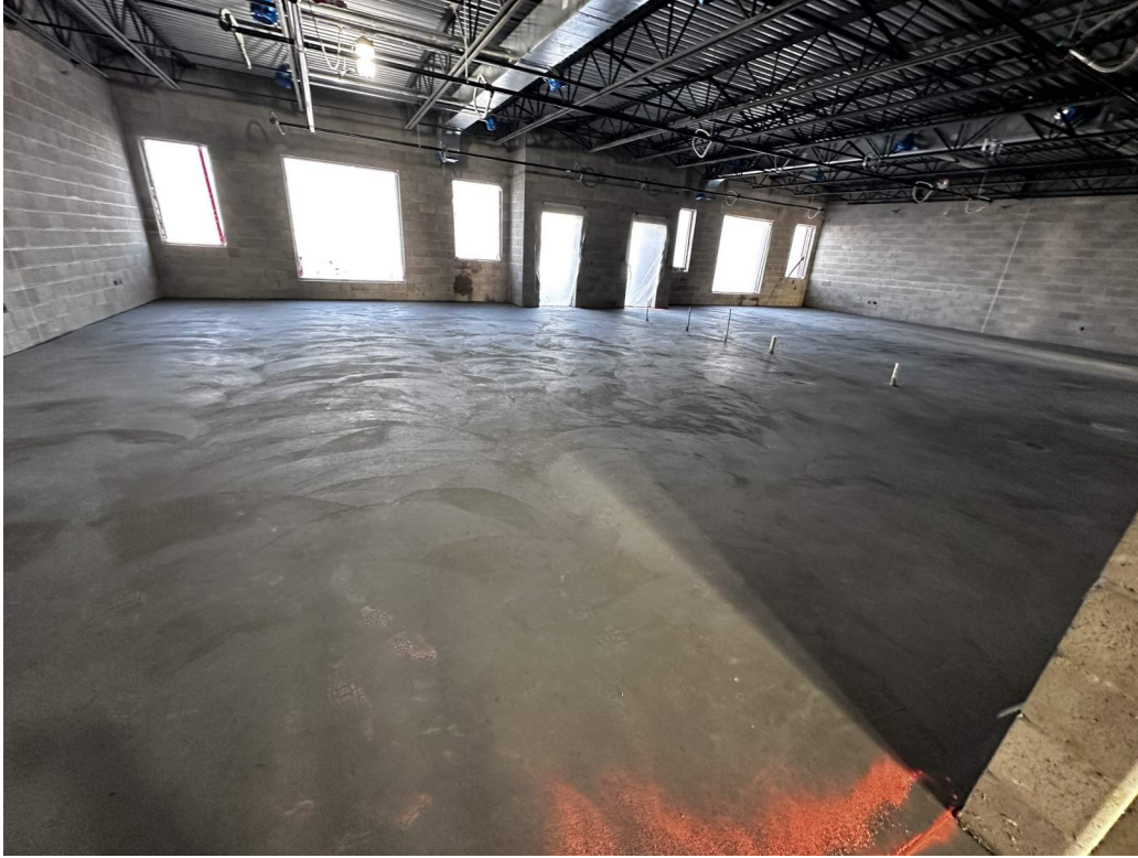
Concrete while curing in a classroom.
