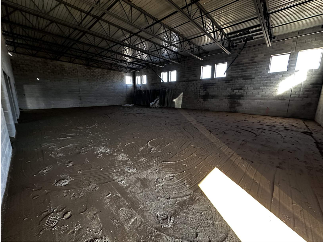
Sand prep prior to concrete in a classroom.
