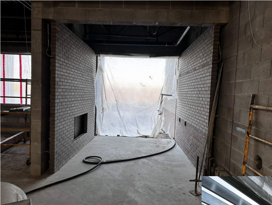
Interior brick veneer at a west side entrance.
