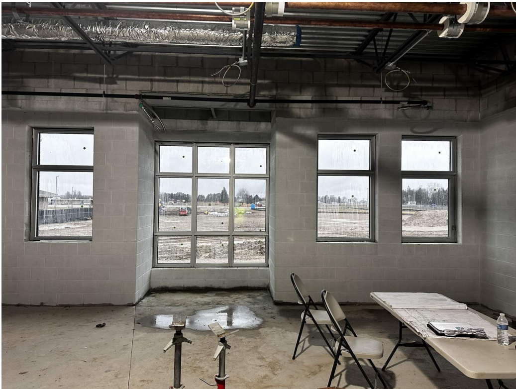
Windows installed and block filler on walls.
