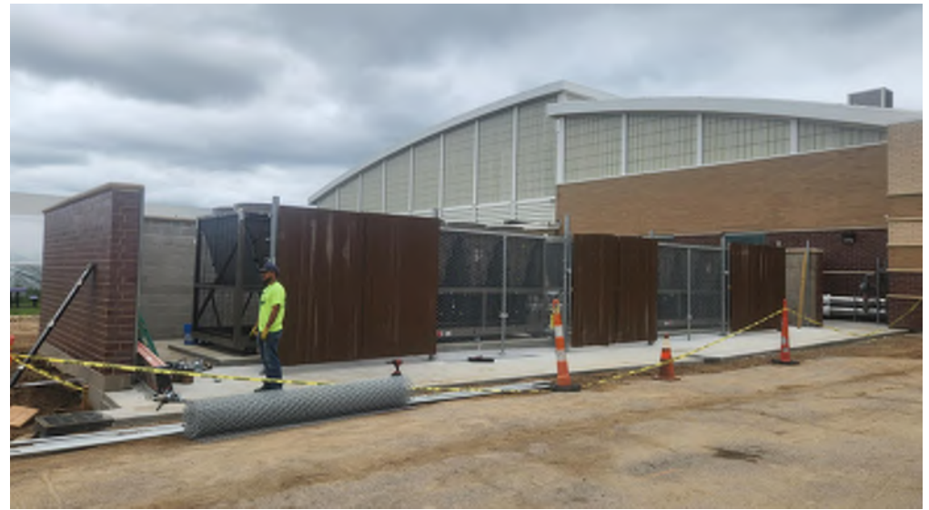
Fencing fabric install in progress at chiller enclosure.
