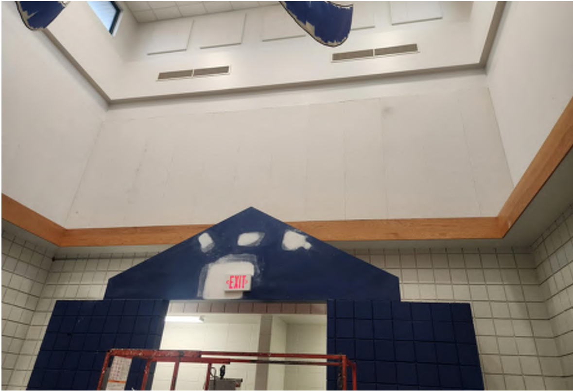
Panels re-installed after mechanical mezzanine work.
