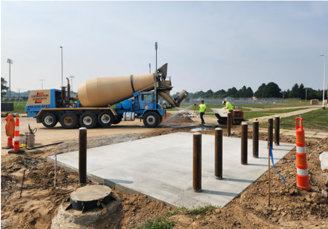
Dumpster pad concrete installed.
