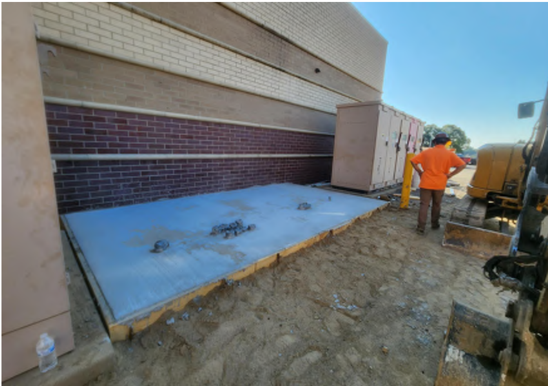
Transformer pad installed on south side of building.
