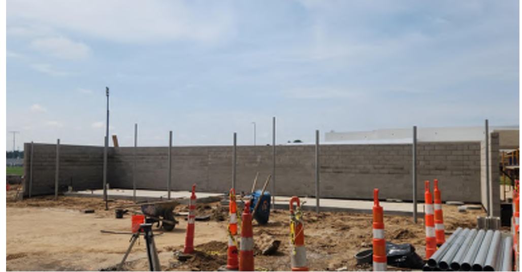
Fencing posts installed at chiller enclosure.
