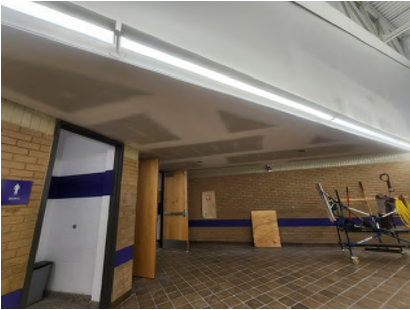
New drywall ceiling before finishing and paint.
