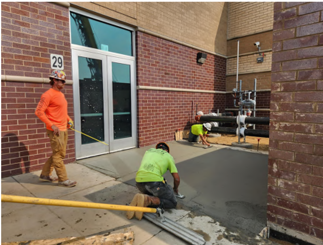
Concrete install near chiller enclosure.
