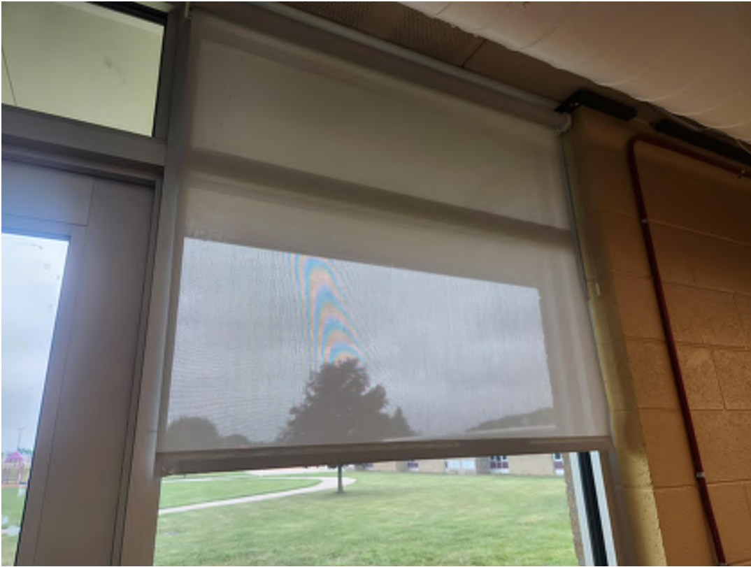
Window shade installed at one of the new classroom storefronts.
