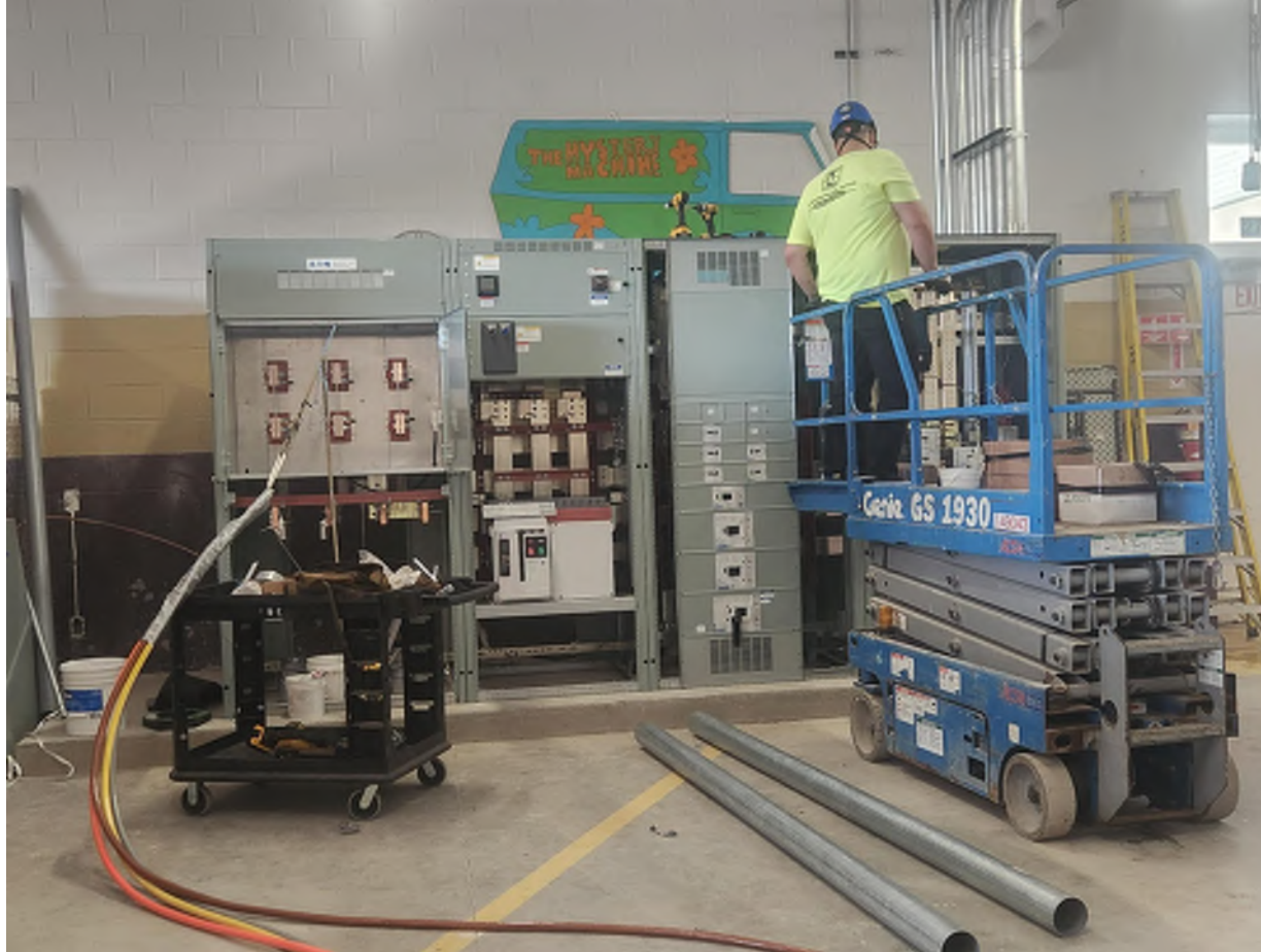
Conduit install at new switchgear in preparation for wire pulling.
