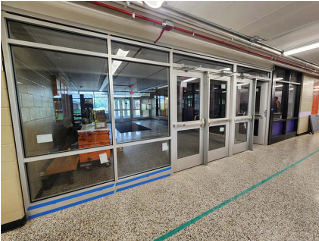
Secure vestibule storefront installed.
