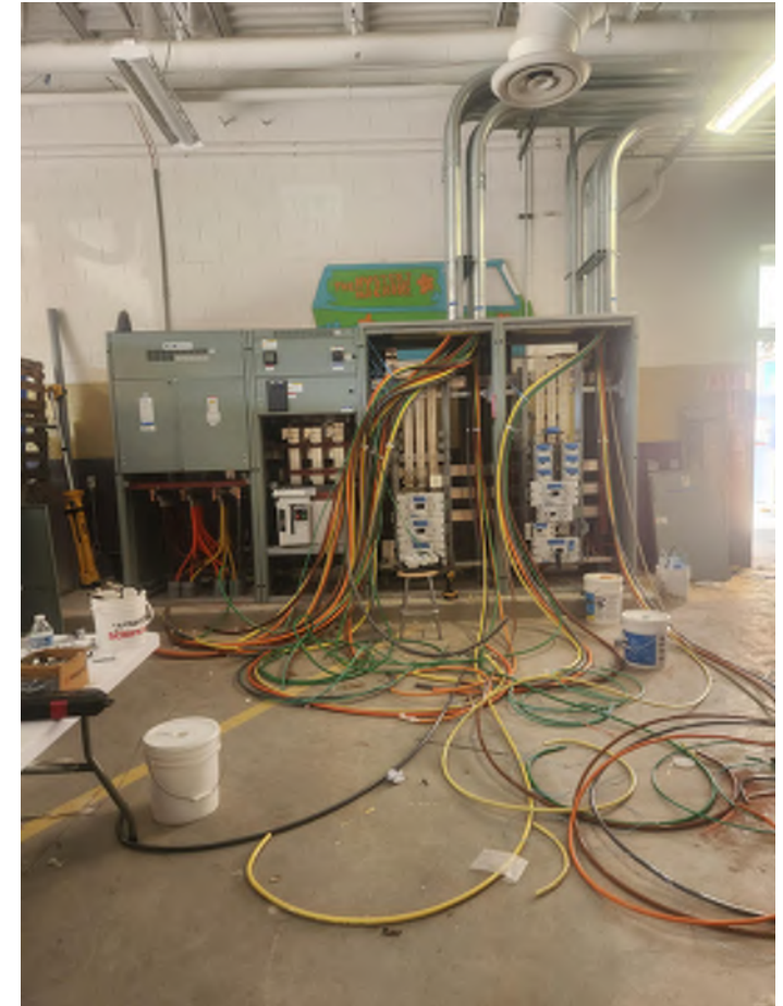
Wire being pulled to new switchgear.
