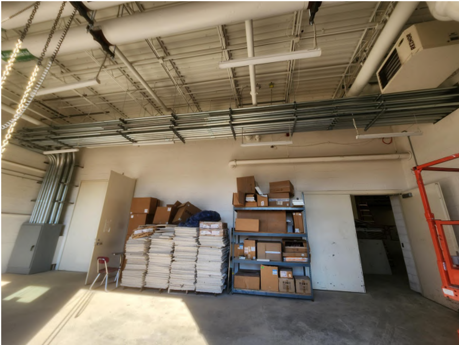
Conduit installed in receiving area for wire to new switchgear.
