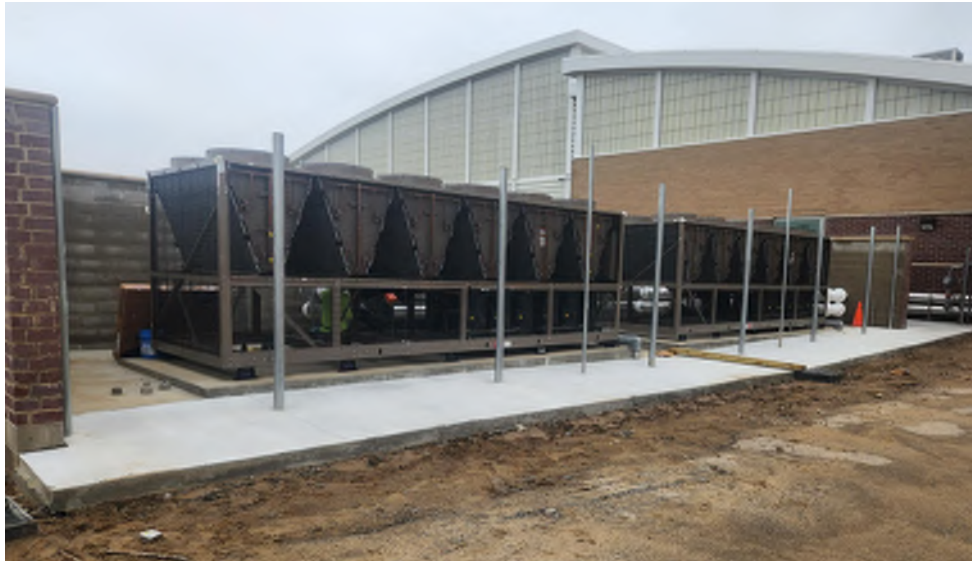
Chillers set and concrete poured in front of chiller enclosure.
