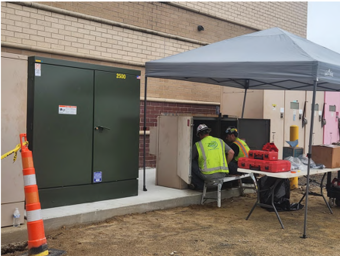
New transformer set on concrete pad.
