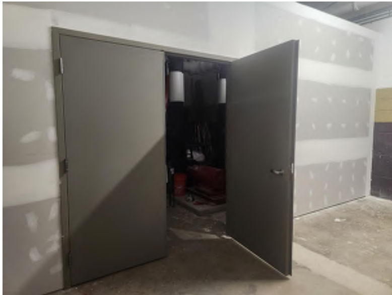
Door installed and wall taped and mudded at pump area separation wall.
