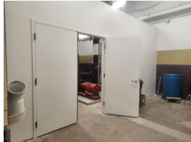
Pump area separation wall finished and painted.
