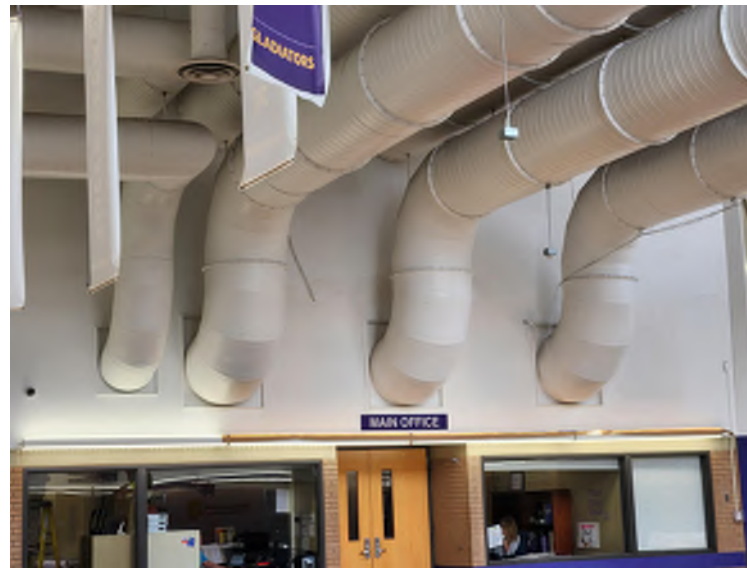
Duct penetrations in filled with drywall and finished.
