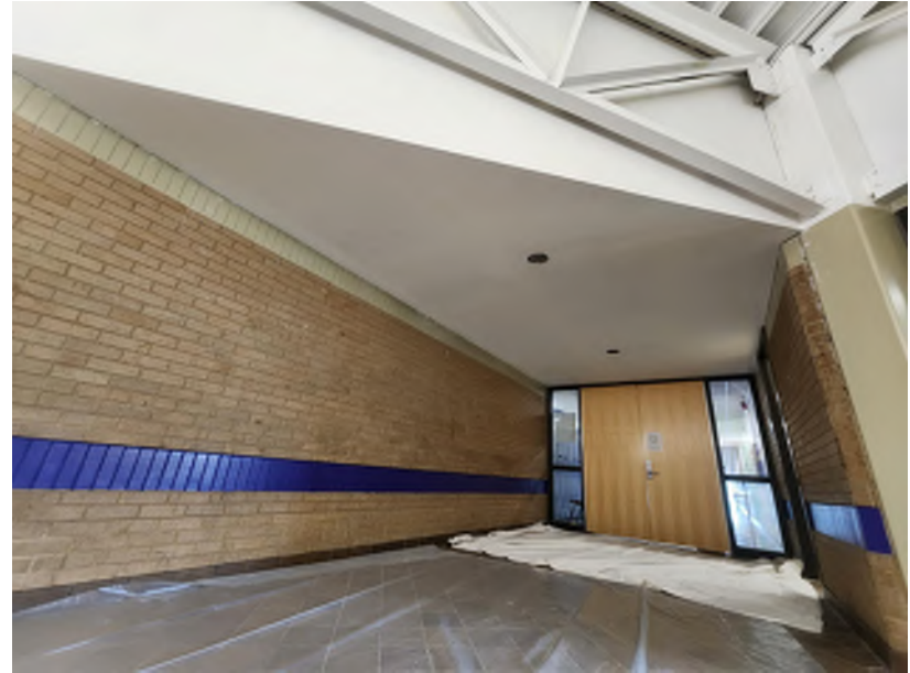
New drywall ceiling after finishing and paint.
