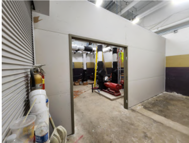
Drywall and door frame installed at pump area separation wall.
