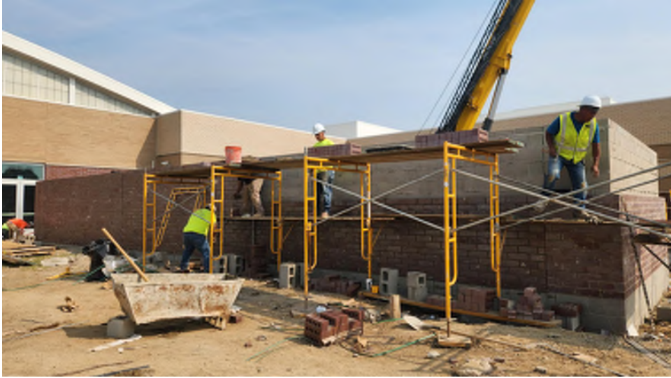
Chiller enclosure masonry in progress.
