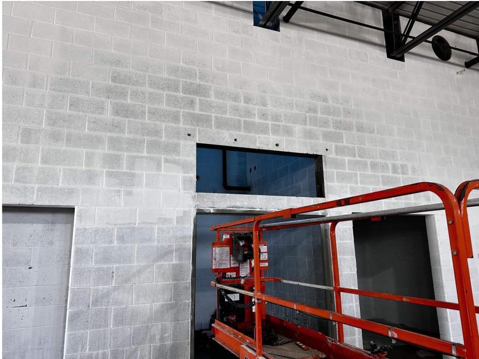
Masonry wall opening after being cut above doorway in the gym.
