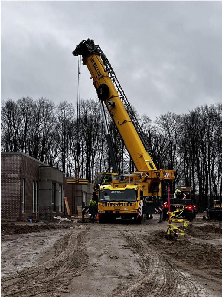
Crane used for RTU lift onto roof.
