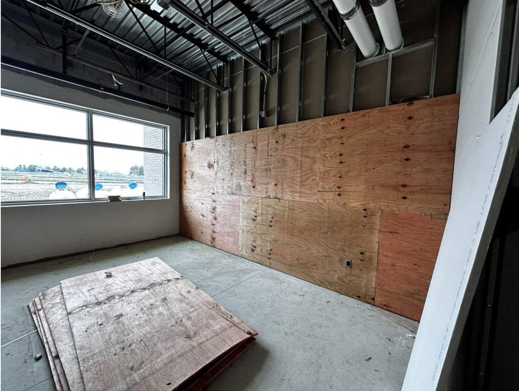
Plywood install in progress in one of the intervention rooms.
