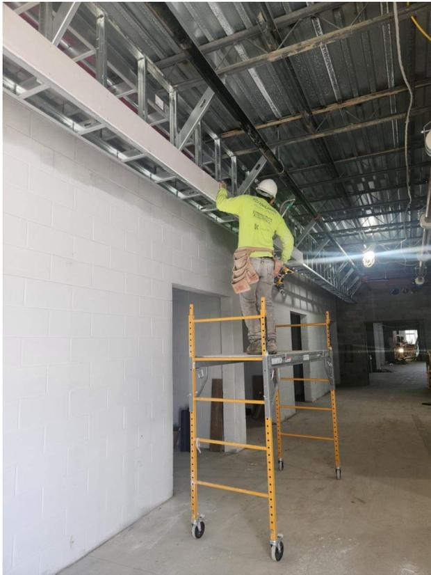
Drywall install at corridor soffit.
