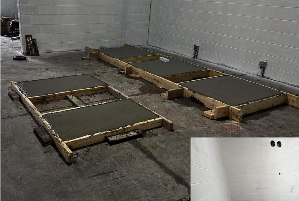
Concrete pads formed and poured in mechanical room.
