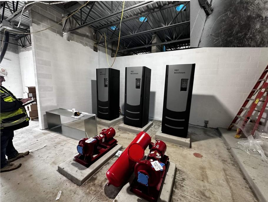
Boilers and pumps installed on concrete pads.
