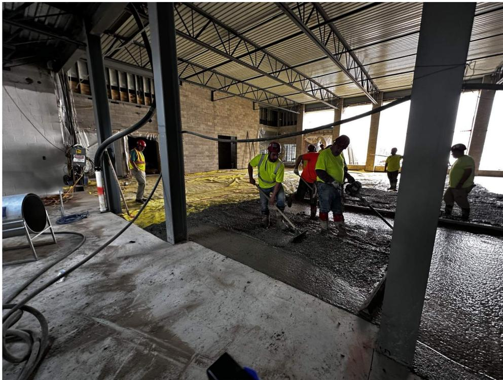
Concrete being spread in cafeteria. All concrete floors have been poured.
