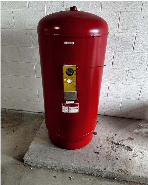
Expansion tank on concrete pad in mechanical room.
