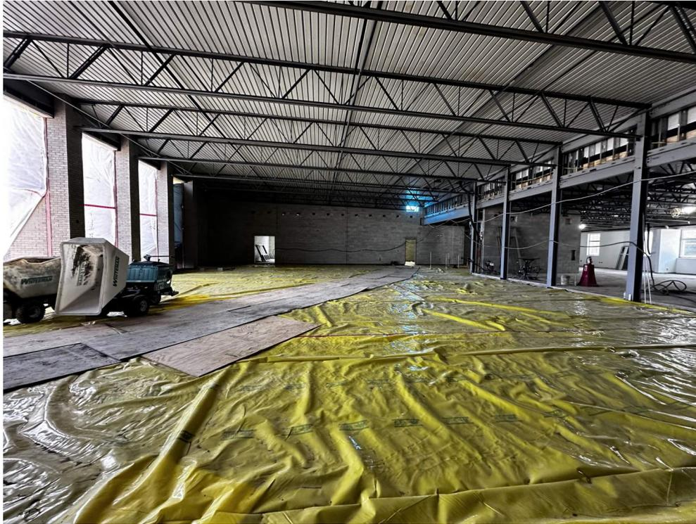
Vapor barrier installed in cafeteria prior to concrete pour.
