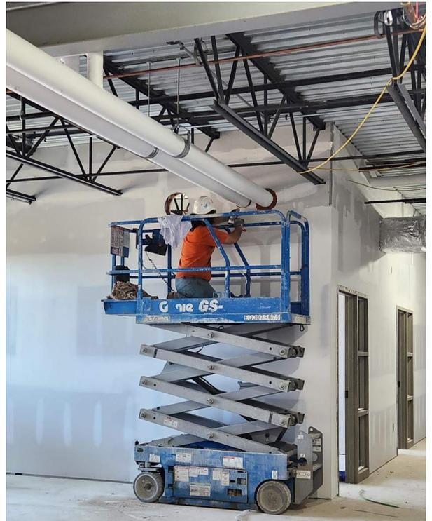
Fire caulking at wall penetration in hallway.
