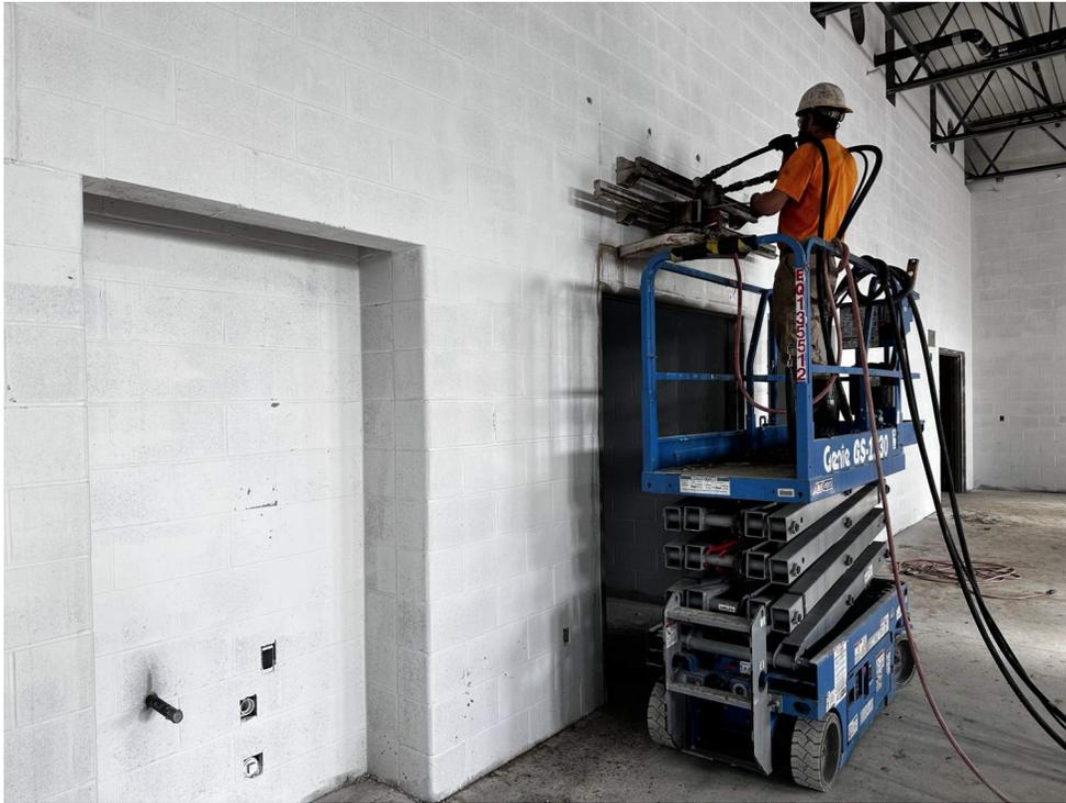
Masonry wall opening being cut above doorway in the gym.
