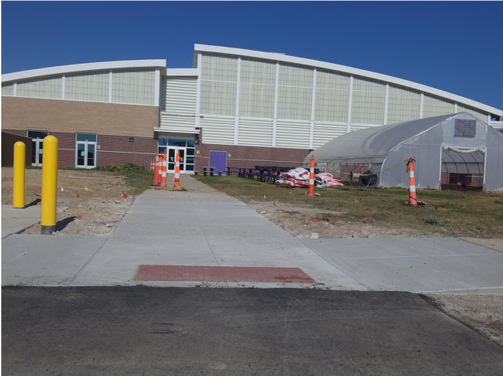
Completed concrete near the dumpster pad.
