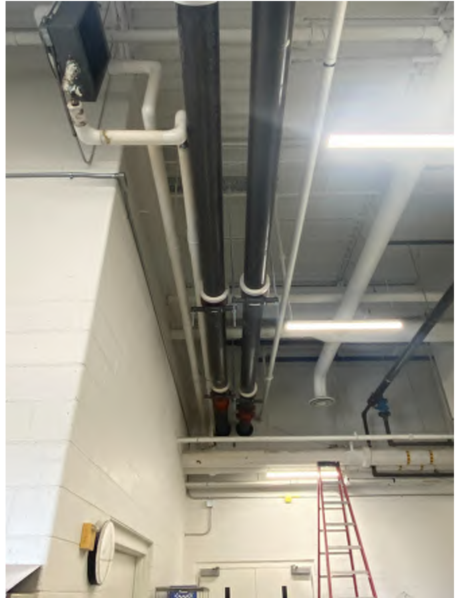
Wall penetrations for piping in receiving area.
