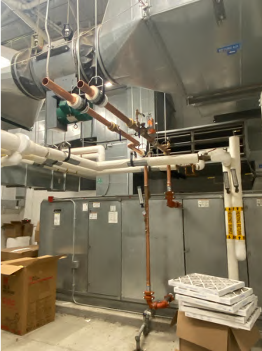
Copper piping in progress in a mechanical room.
