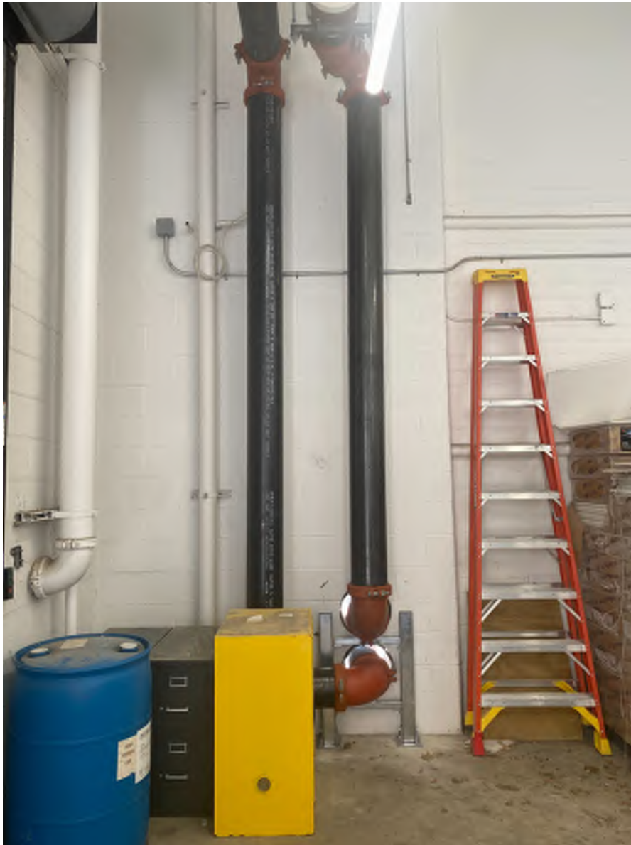
Wall penetrations for piping in receiving area.
