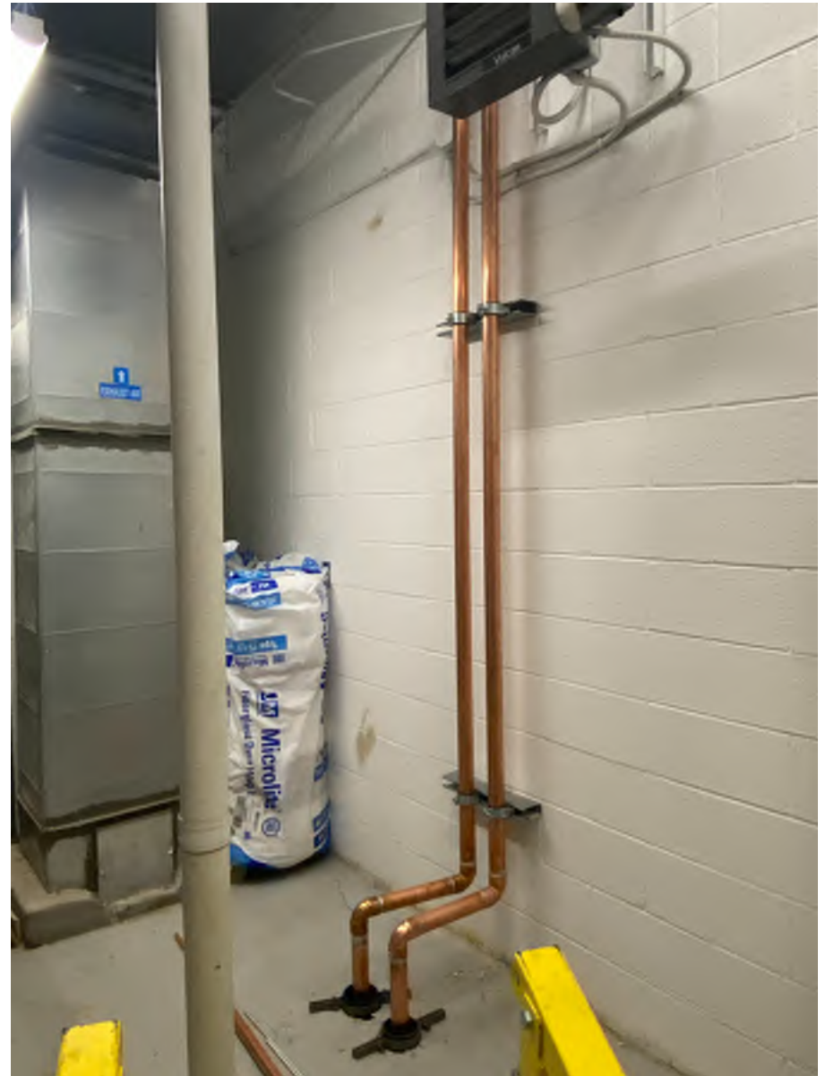
Copper piping in progress in a mechanical room.
