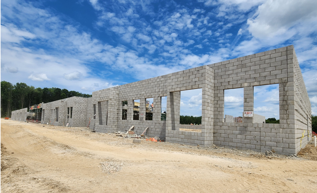
Exterior view of masonry walls at south west corner of building.
