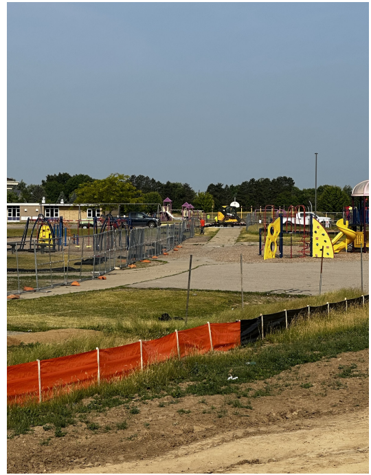
Fencing moved to include Kreeger playgrounds that will be replaced.
