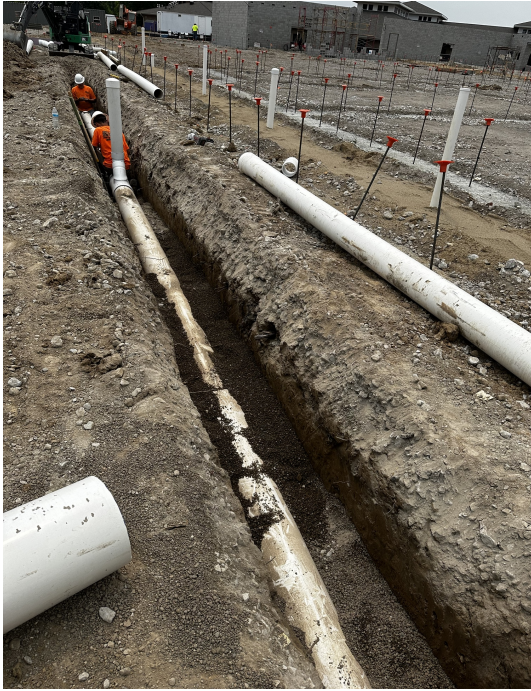
Plumbing pipe install within open trench.
