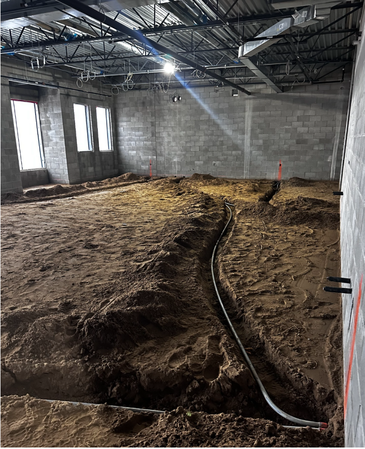
Underground conduit in progress.
