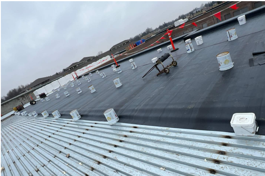
Roofing in progress and warning lines installed.
