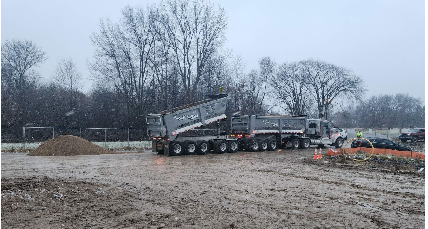
Sand being delivered to job site for interior flatwork.
