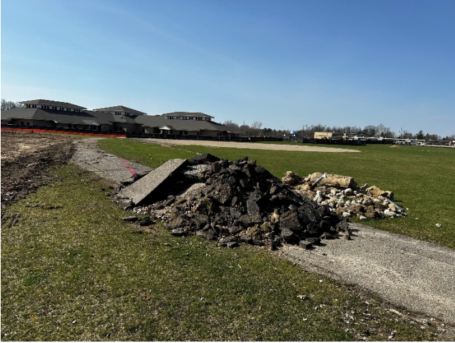
Asphalt removal at west side of site (complete).
