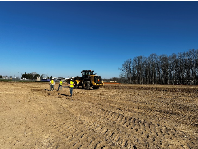
Proof roll of building pad (complete).
