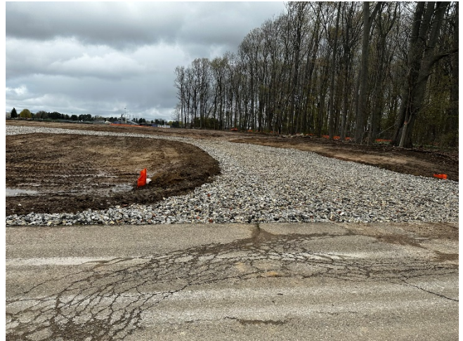
Install of stone access road and material staging areas (ongoing).
