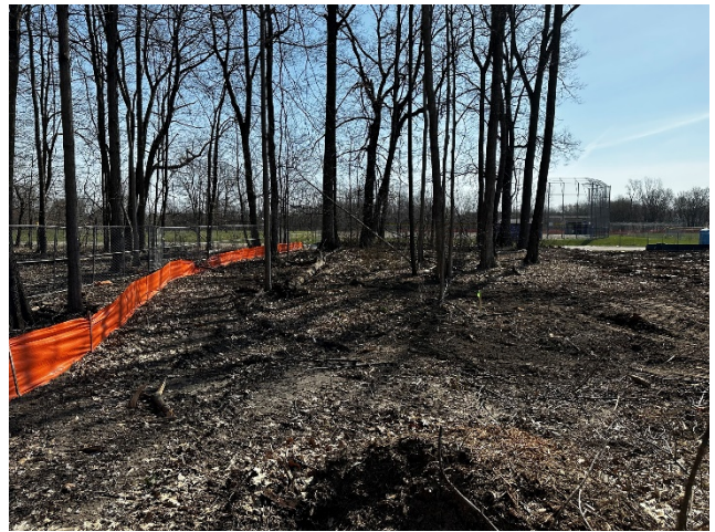
Trees removed on east side of site due to instability (complete).
